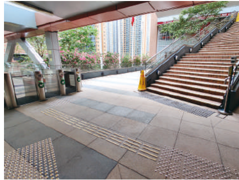
A new tactile guide path is installed on the PolyU HHB Campus. 理大紅磡灣校園鋪設了新的觸覺引路帶。
